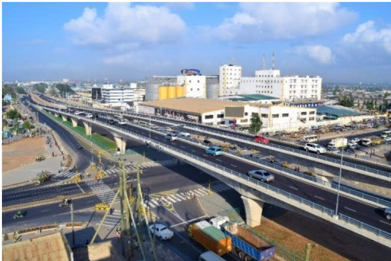
(Photo) Completed Tazara intersection (Courtesy of Sumitomo Mitsui Construction)
