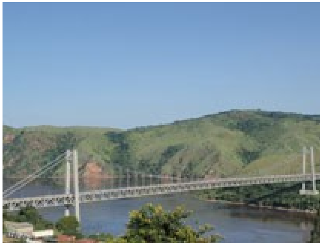
Matadi Bridge (photo cited from JICA)
