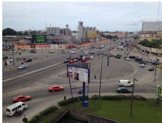
Before construction (Courtesy of the JICA webpage)
